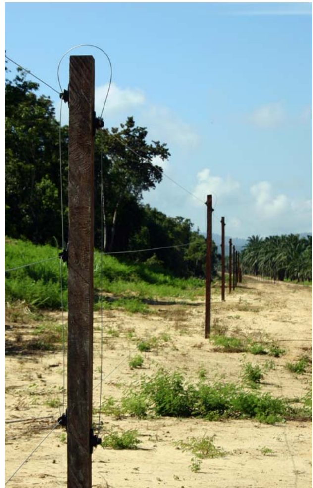
Figure 6. A three-strand electric fence with the posts wired.
