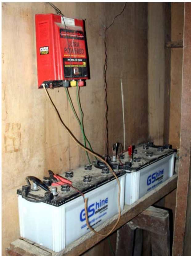
Figure 7. An energizer powered by wet-cell batteries.
